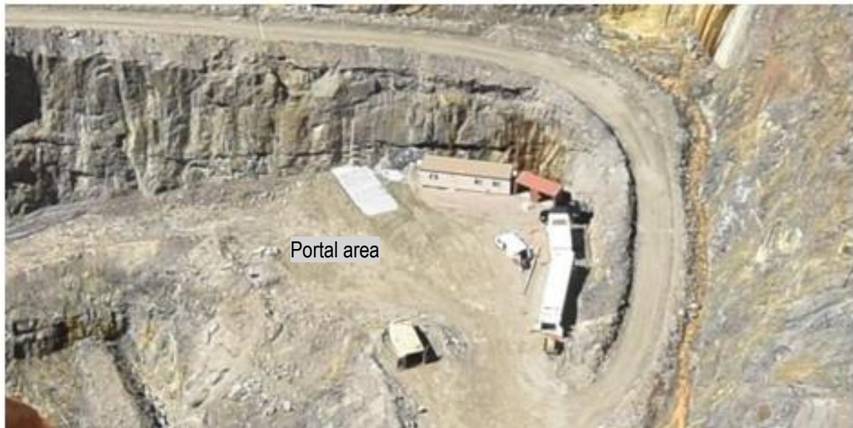
Figure 5 Preparing for the commencement of the underground portal and decline
