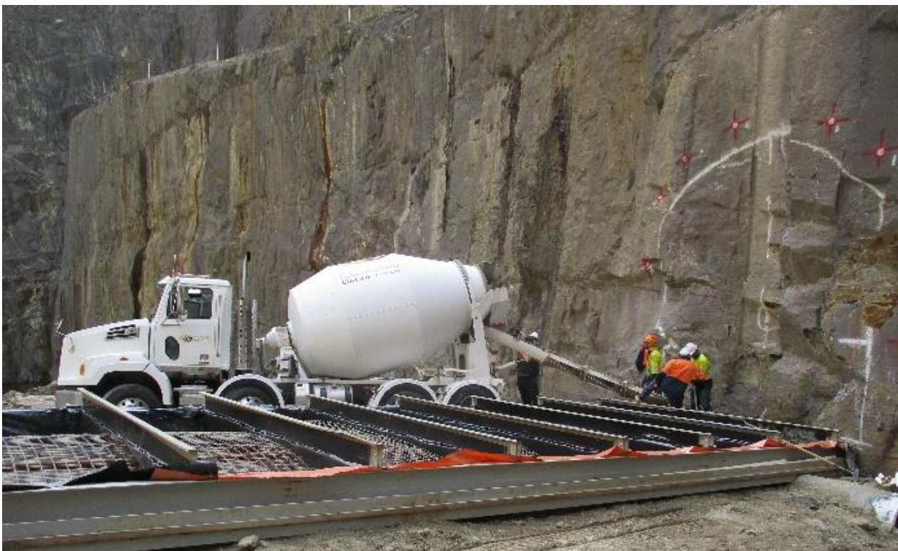
Figure 5 Preparing portal for Komatsu MC51
