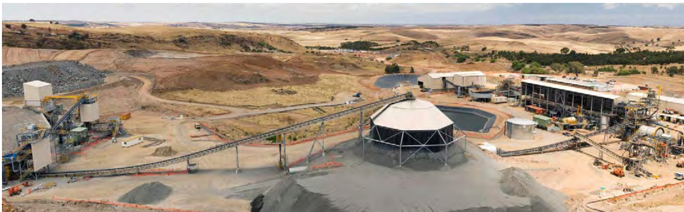
Foreground: Crushed low-grade ore stockpiled adjacent to the live stockpile under the dust containment cone
