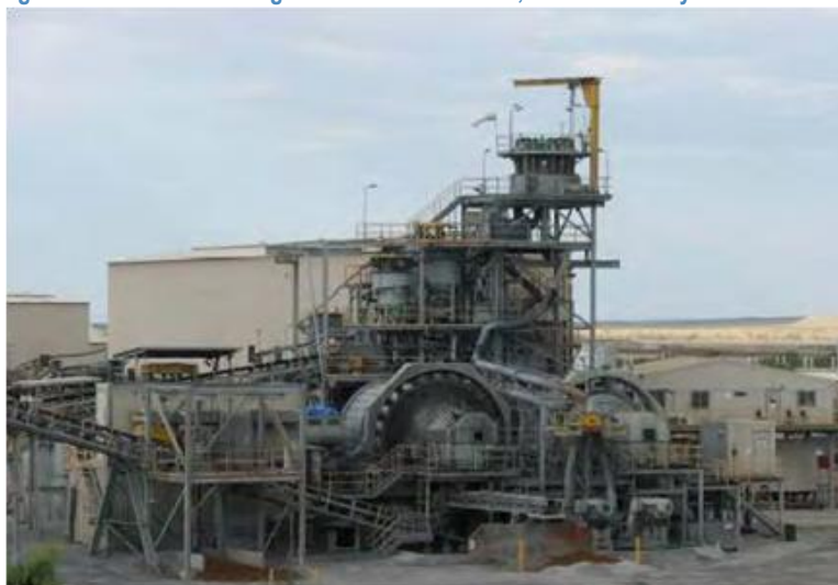
Figure 3: Pillara Processing Plant at Lennard Shelf, Pre Removal by HGO
