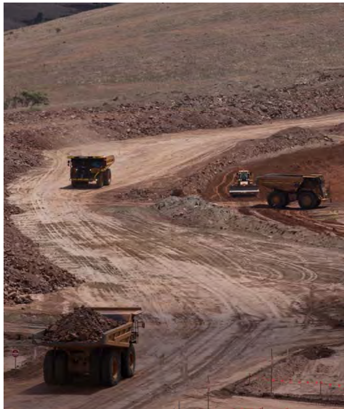
Plate 1. TSF Embankments Being Constructed
