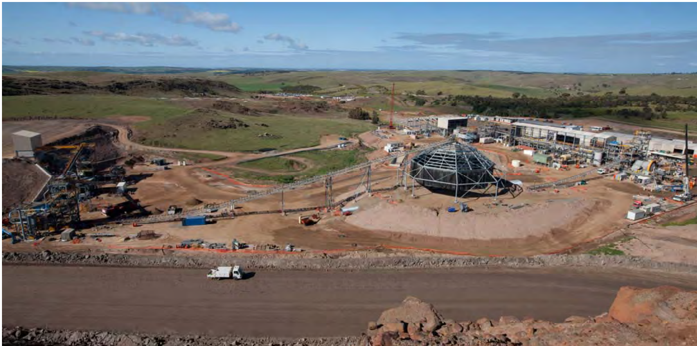
Plate 1. Processing Plant Construction Area, Kanmantoo Copper Mine (30/8/11)
