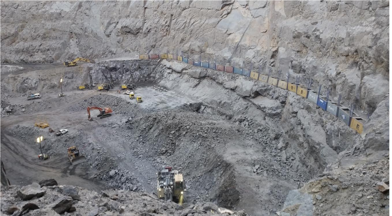
FIGURE 2. ROCK CATCH FENCE CONSTRUCTED USING SEA CONTAINERS
