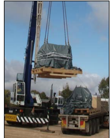
Arrival of new equipment at the Kanmantoo Site
