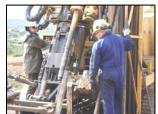
Contractor operating drill rig
