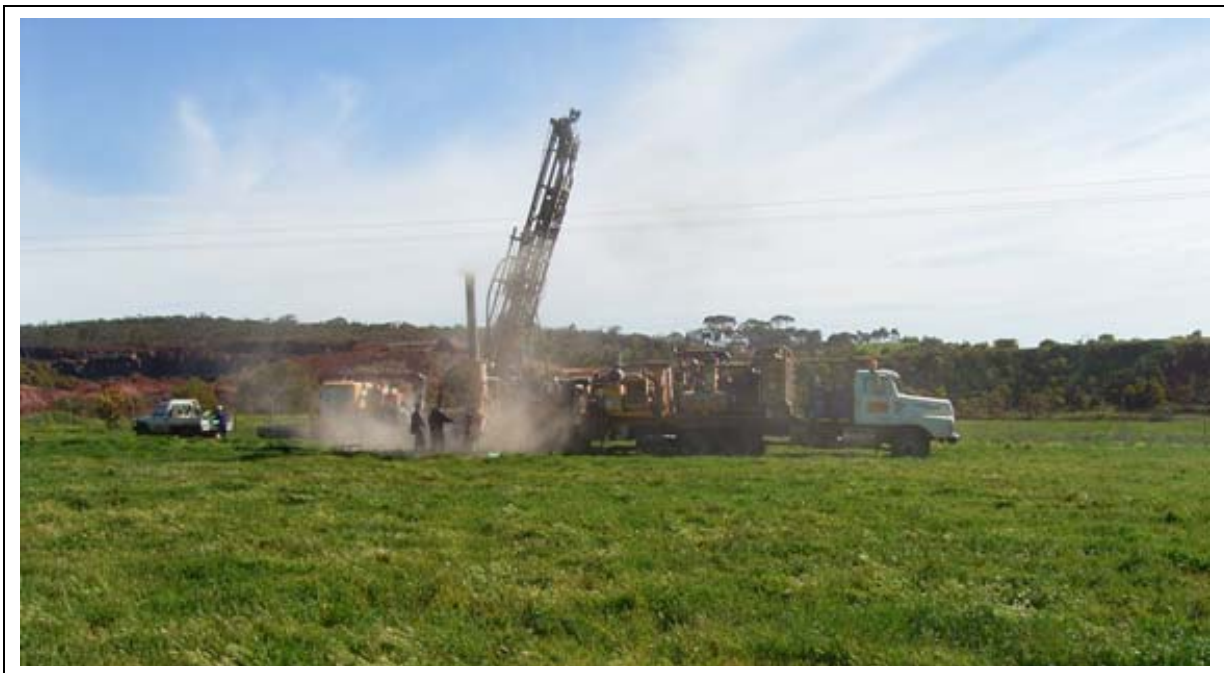
RC Drilling at the old Kanmantoo mine
